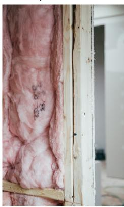
Any type of insulation will theoretically be ecofriendly if it sufficiently cuts down on energy used for heating and cooling. However, some of this saving is negated if batts, fillers, and/or sprays used for insulation are not sustainably sourced or use toxic chemicals to help in binding and fire resistance.
